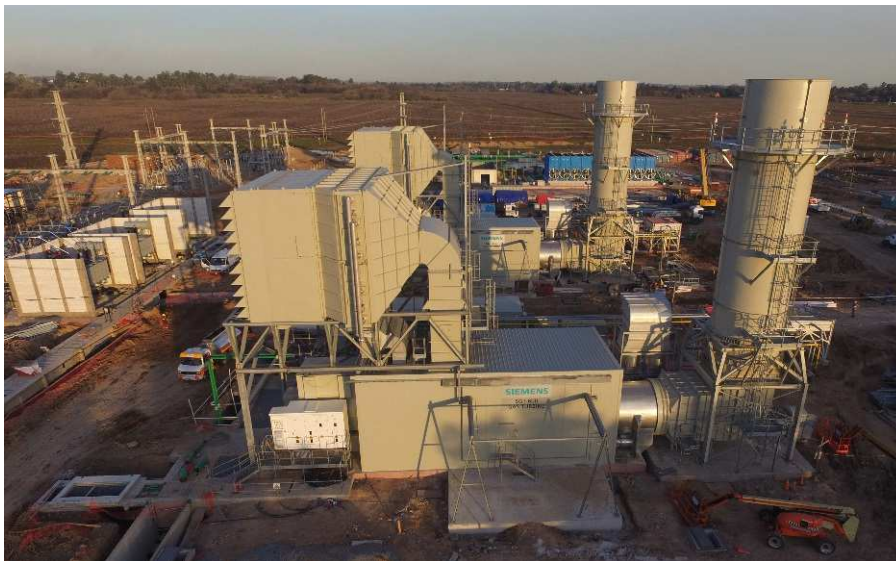
07/26/17 – Turbines installed
