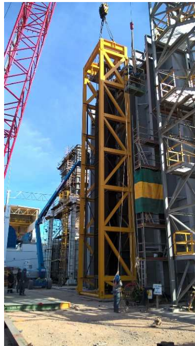
08/05/17 - Assembly of boiler decks
