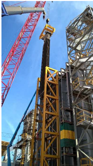
08/05/17 - Assembly of boiler decks
