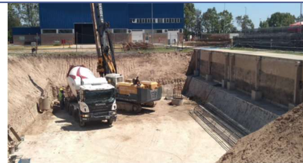
Piloting works for ST6 foundation
