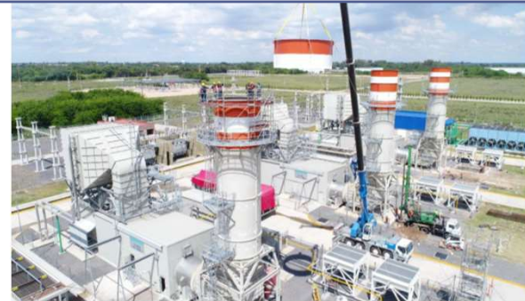
GT3 Chimney extension already executed
