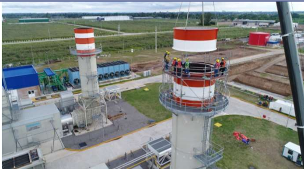
GT2 Chimney extension already executed
