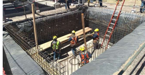
Excavation for the Blowdown tank
