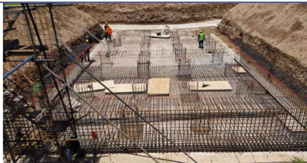
Assembly of the armors for ST5 foundation
