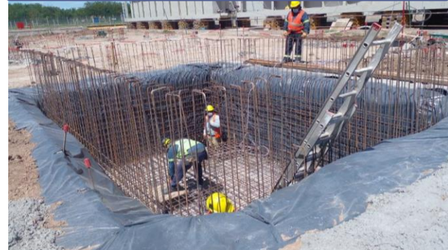
Purge tank foundation
