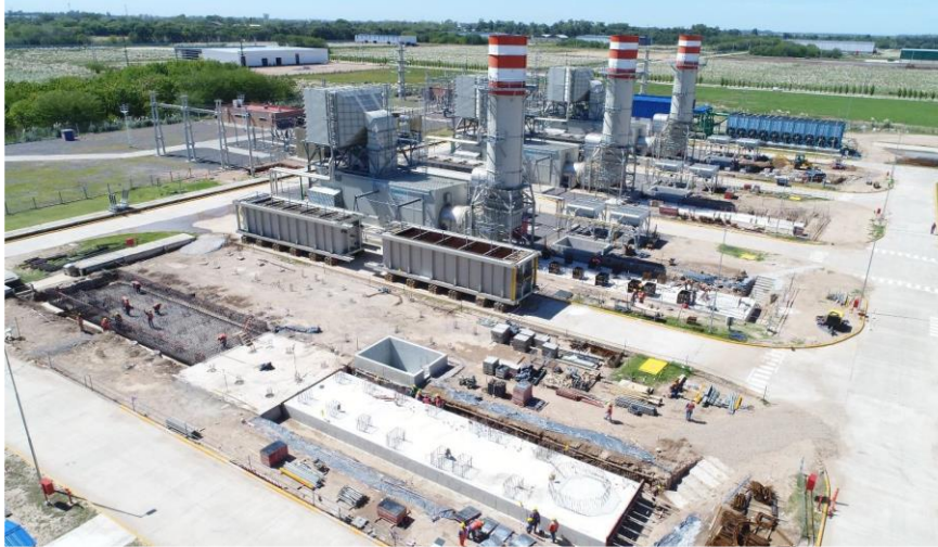
Concreting of GT4 and Boiler Foundations
