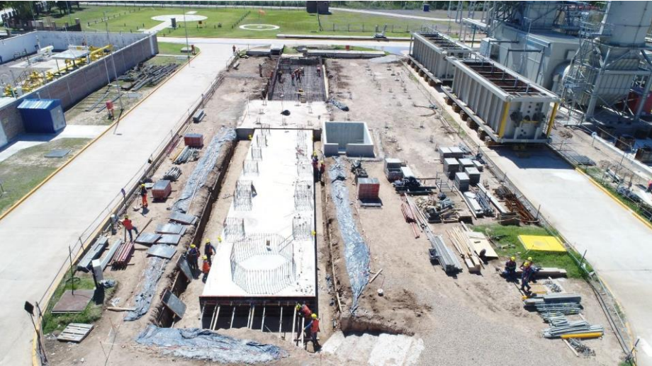
Concreting of GT4 and Boiler Foundations
