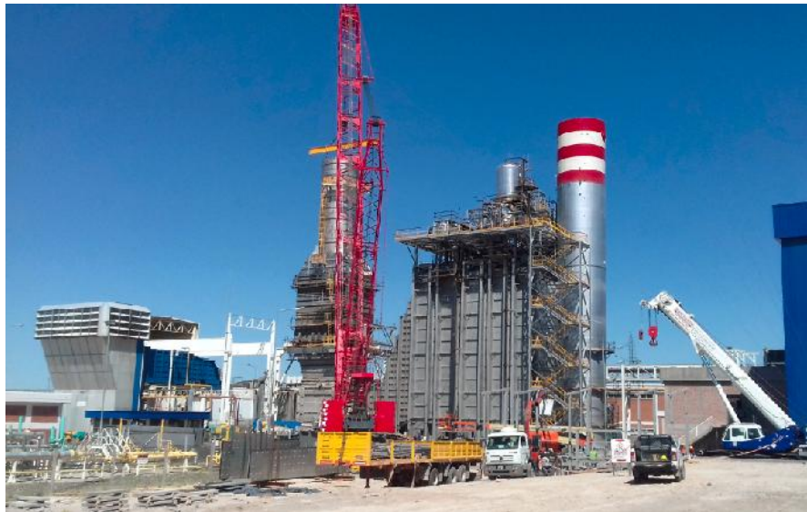
02/09/18 – Chimney by pass assembly
