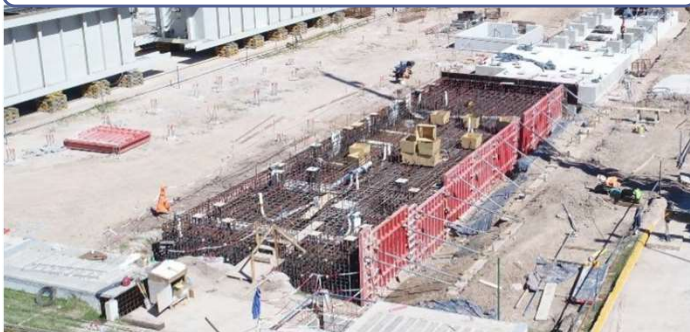
Assembly of the armors for GT4
