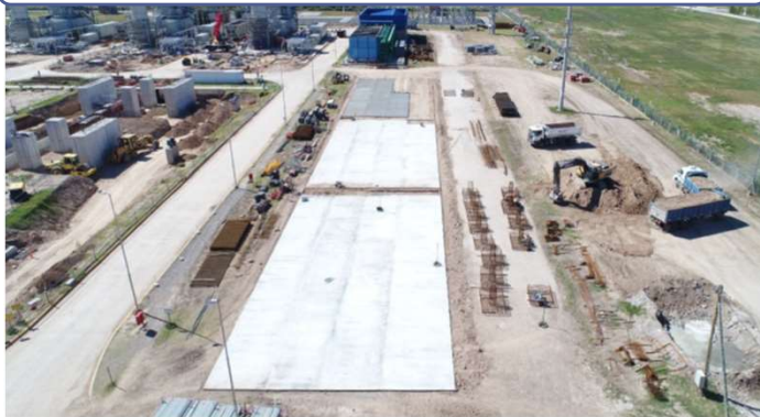
Assembly of the armors for GT4
